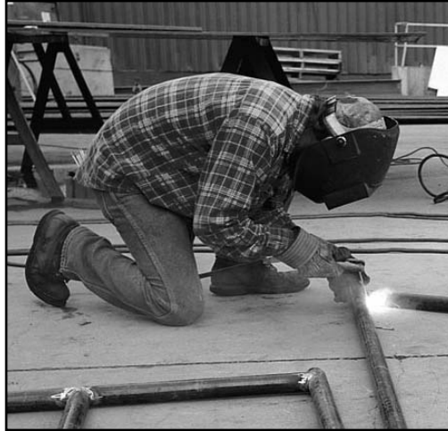
Stick Welding Application
