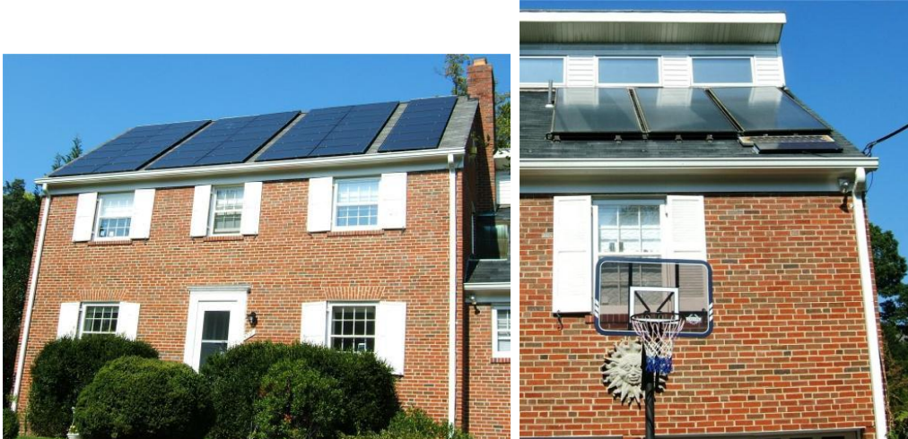
This Bethesda, MD home has photovoltaic panels in front and solar collectors in the rear for heating the family's water. Photos by author.
