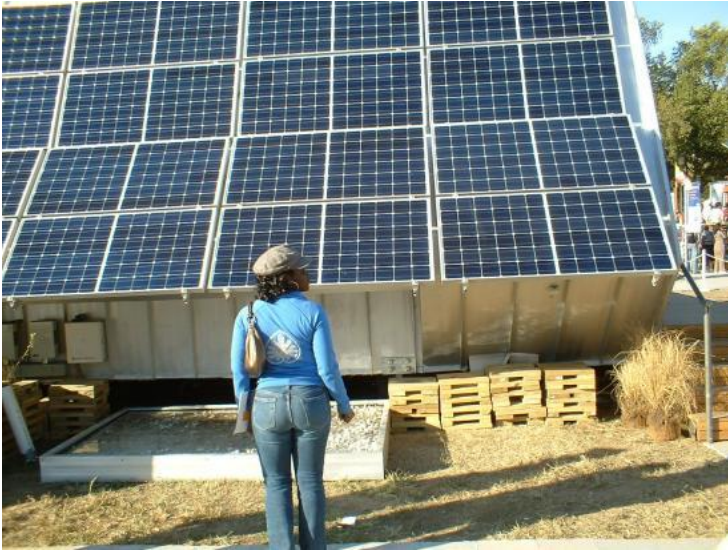
This PV array has one onlooker gazing upward in awe. 2007 Solar Decathlon, Washington, DC. Photo by author.
